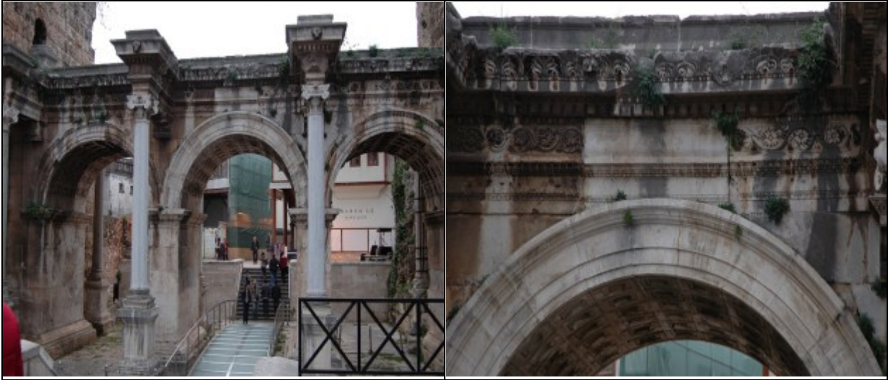
Figure 9. Hadrian's Gate, also known as Üçkapılar, and its arch detail. Photo by Nurdan Akiner.
